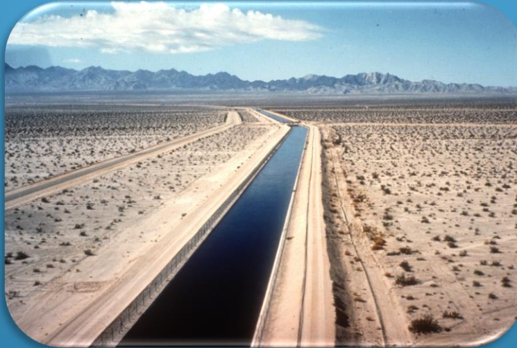
Colorado River Aqueduct 5 Pump Stations 493 m lift (1,617 ft.)
